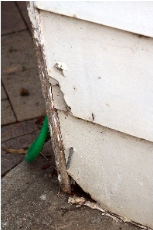
Asbestos Location - broken cladding_5973.jpgg
