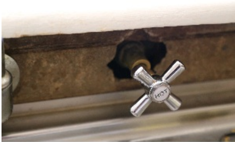
Unpainted Damaged Asbestos Cement Splashback 046.JPG
