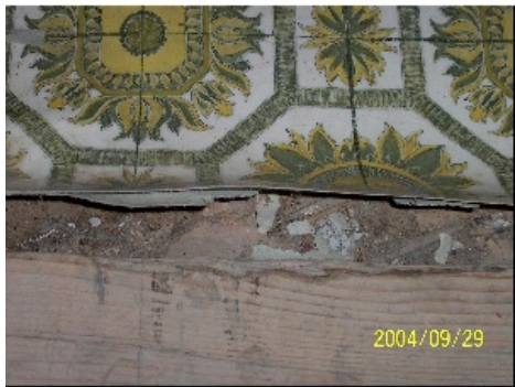
asbestos paper under lino.jpg
