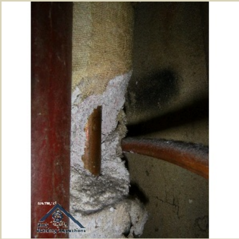
Pipe lagging service cupboard2.jpg
