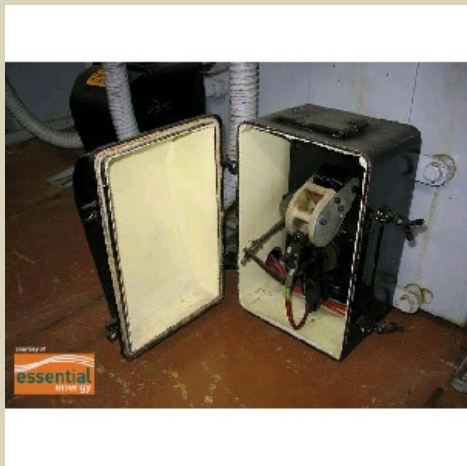
Oil Circuit Breaker Closing Contactors.jpg
