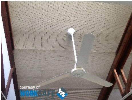
WA DptCom_Low density fibreboard ceiling panels chrysotile and amosite_0182.jpg
