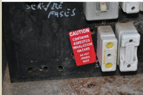
114 Asbestos Power Boards_.jpg
