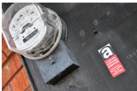
0116 Asbestos Power Boards_.jpg
