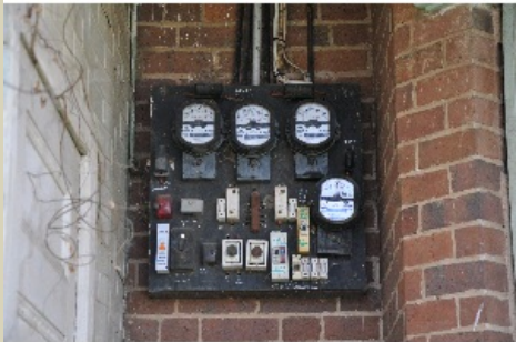
108 Asbestos Power Boards_.jpg
