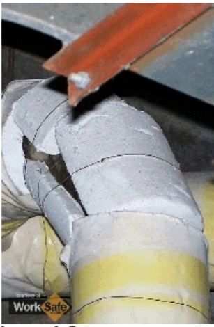
WST_formed-flue-pipes-incorrectly-tied-back.jpg
