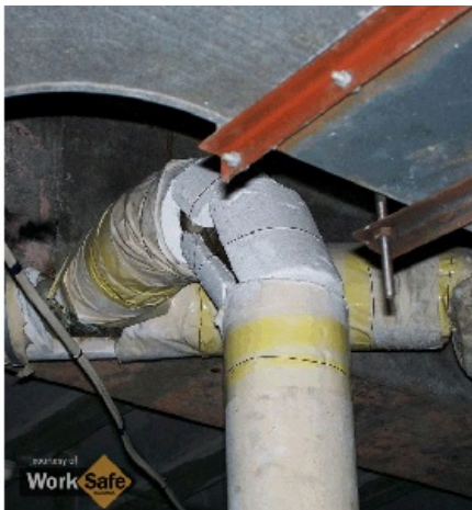
WST_asbestos-containing-formed-flue-pipes.jpg
