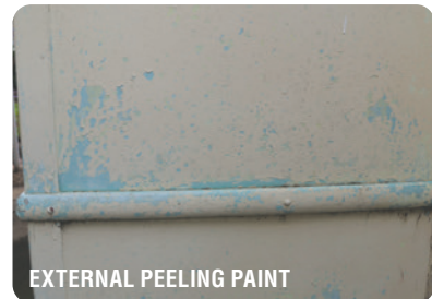
PEELING PAINT, EAVES, GUTTERING AND DOWNPIPE
