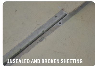
BROKEN ASBESTOS CEMENT SHEETING
