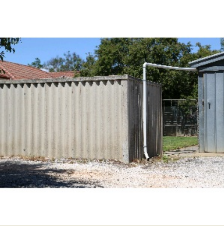
Fencing with capping 2527 Courtesy of Asbestos Awareness.JPG
