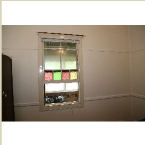
Asbestos Cement Walls_0296.JPG
