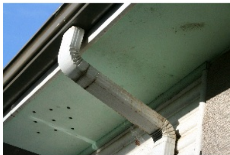
guttering and eaves_5971.jpg
