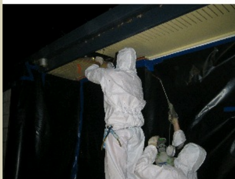
Soffit - eave removal.jpg
