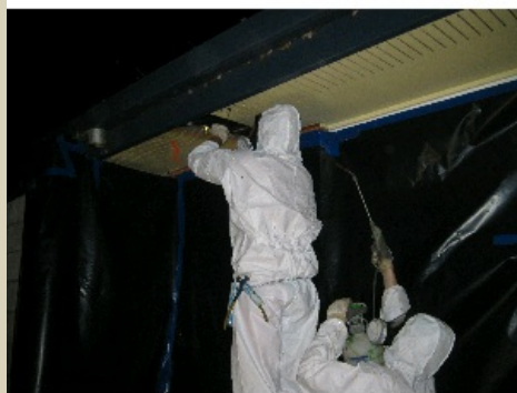
Soffit - eave removal.jpg
