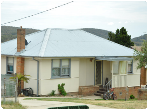
CORRUGATED ASBESTOS ROOFING AND FLUE
