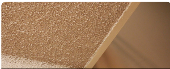
VERMICULITE CEILING OFTEN IN APARTMENTS
