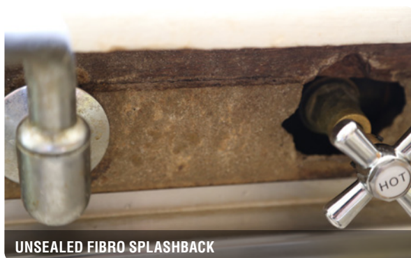
UNDER KITCHEN SINK. UNSEALED FIRBO WALL & AROUND PLUMBING
