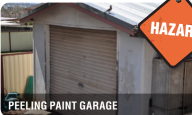
EXTERNAL PEELING PAINT ON AC WALL
