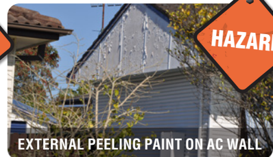
EXTERNAL PEELING PAINT ON AC WALL
