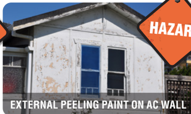
EXTERNAL PEELING PAINT ON AC WALL
