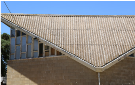
Asbestos Cement Roof
