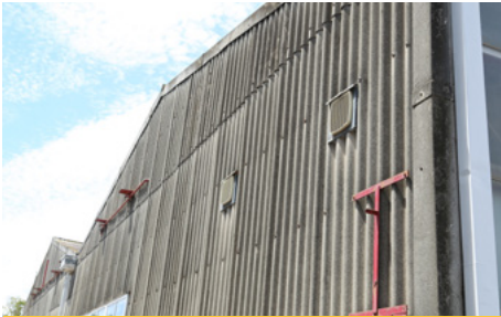
AC Cladding, Flashing & Capping
