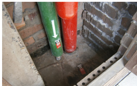
Asbestos Cement & AC Pipes
