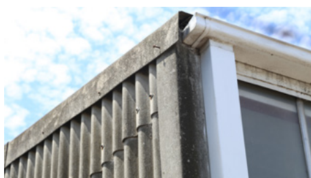
Wall Cladding, Flashing and Corner Capping
