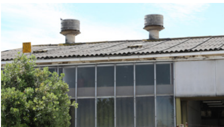
Flue, AC Roofing, Ridge Capping and Guttering
