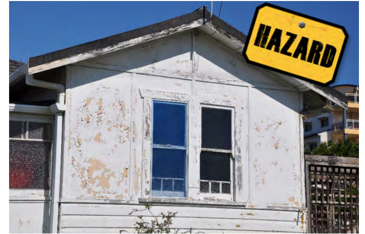
AC Sheeting: Unsealed or left to weather, bonded asbestos will become friable. Image: Asbestos Awareness
