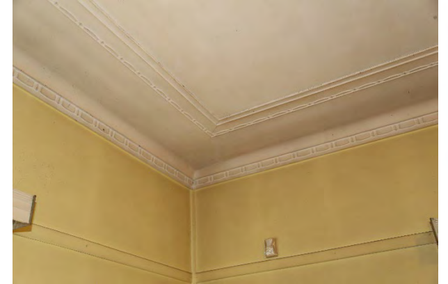
Non-friable: Residential AC sheeting and moulded joining strips
