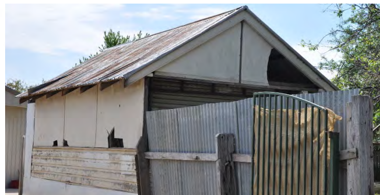
Broken & weathered AC sheets
