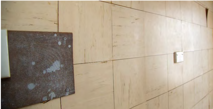
Under lino: glue & backing
