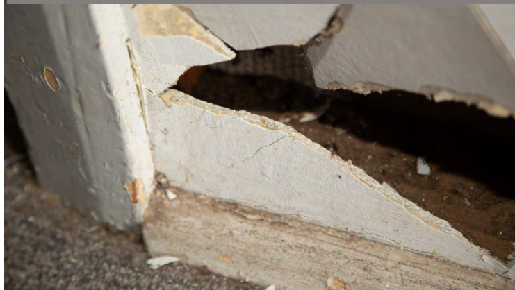
Broken AC Sheets (fibro) Internal
