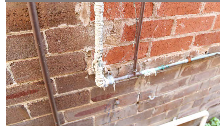
Friable rope around hot water pipe
