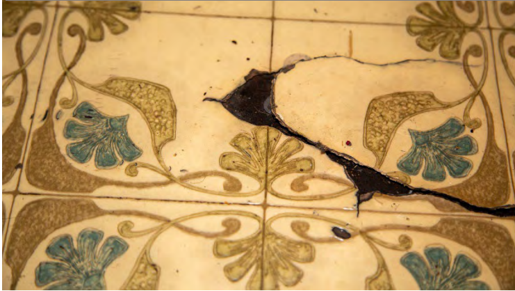
Under vinyl floors: glue & backing
