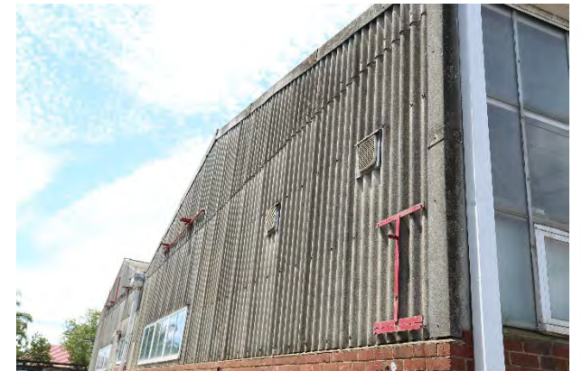
Unsealed: Commercial AC sheeting (exterior), flashing and drain pipes
