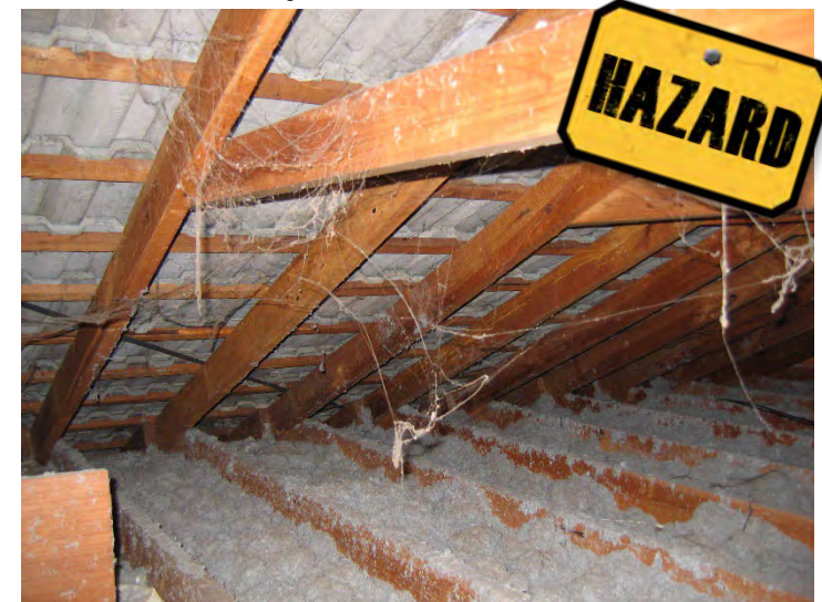
Mr Fluffy: loose fill asbestos insulation
