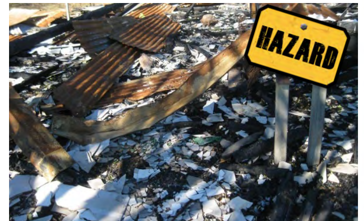
Fire Damaged ACMs Image: Townsville Asbestos
