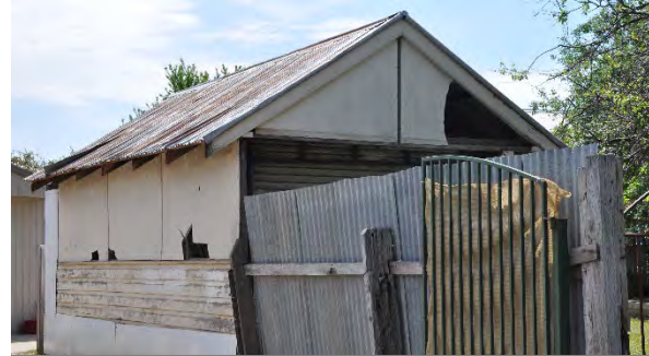
Unsealed & broken AC Sheets
